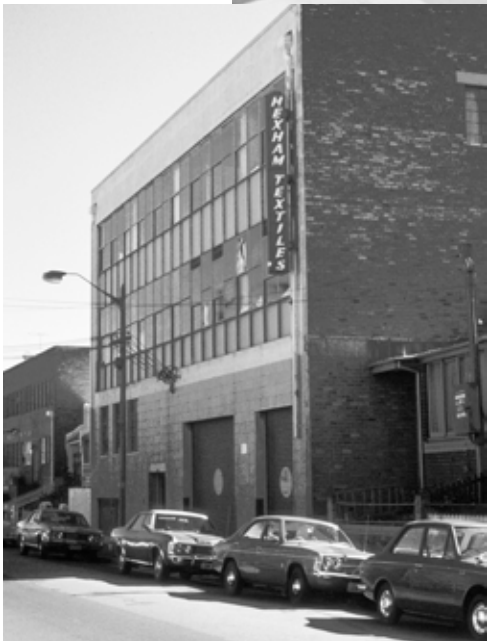
Hexham Textiles building, Rosebery // c1977 (City of Sydney Archives: 057945)
